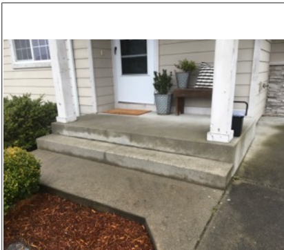
Image of service walk and steps.
