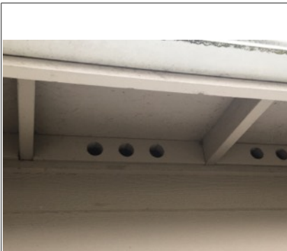
Image of soffit
