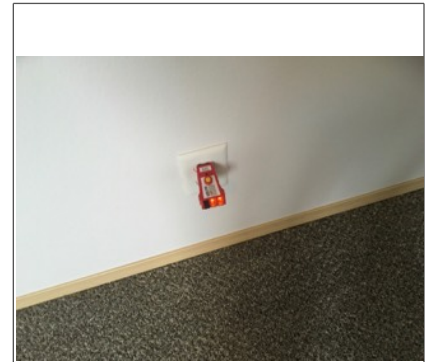
Image of tested electrical outlet
