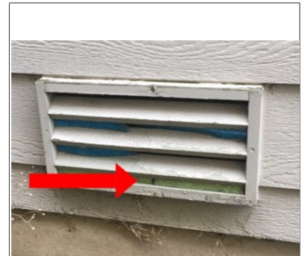
Insulation installed inside louvers of crawl space ventilation.
