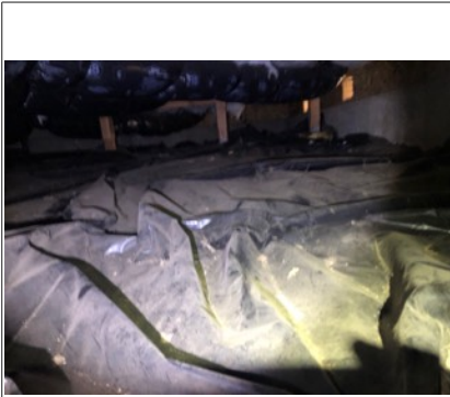
Image of vapor retarder on top of gravel floor
