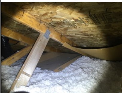
Image of OSB roof sheathing inside attic.
