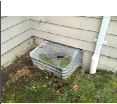
Image of crawlspace access
