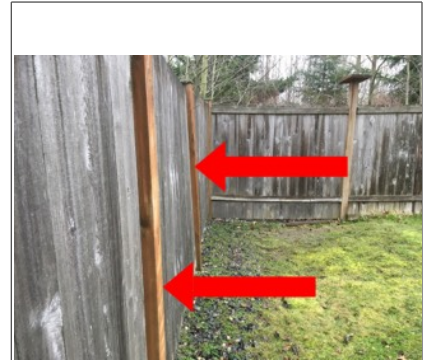
There are several fence posts located in the backyard that are leaning improperly. Recommend further evaluation/repair by licensed fencing contractor.
