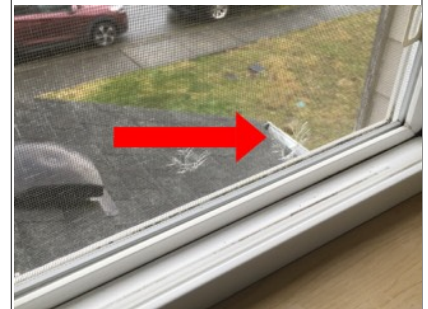
Damaged window screen
