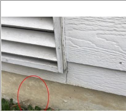
Image of poured concrete foundation.
