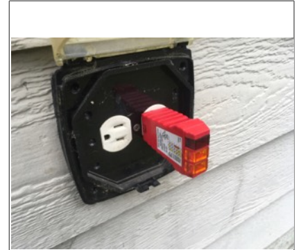
Image of tested outlet on east side of building.
