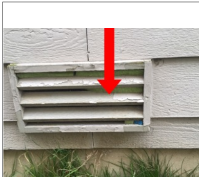
Insulation installed inside louvers of crawl space ventilation.
