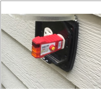
Image of tested outlet on north side of building.
