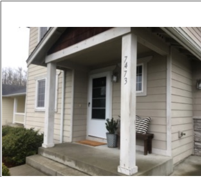
Image of front entry door porch cover.
