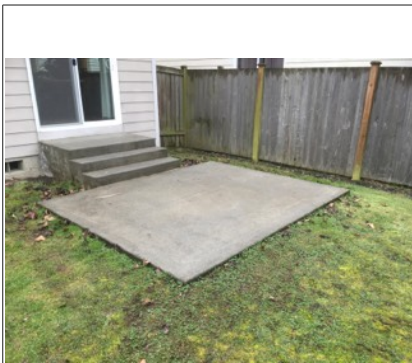
Image of concrete patio
