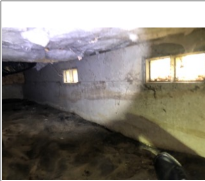
Image of poured concrete foundation walls
