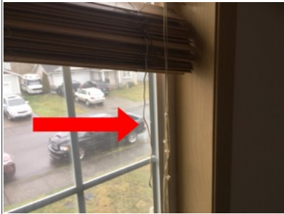
Image of damaged cord on master bedroom blinds.
