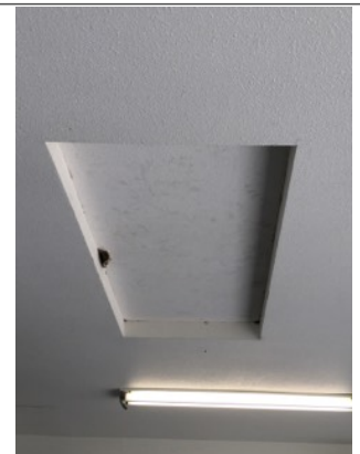
Image of attic hatch in garage
