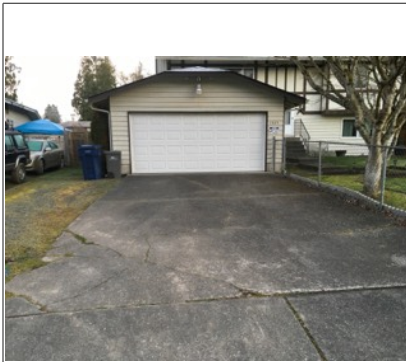
Image of garage door (exterior view)
