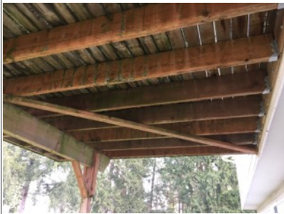
Image of cross-bracing of deck
