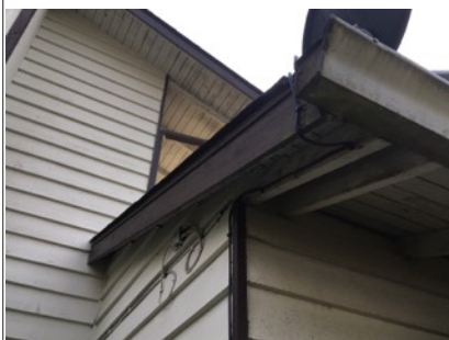
Image of fascia board and metal rake edge trim.
