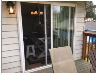
Image of sliding glass door ending to patio.
