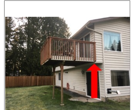
Image of the cantilevered deck attached to the cantilevered section of the house. See statement.
