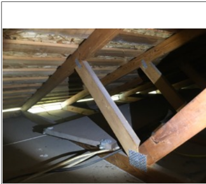
Image of roof truss
