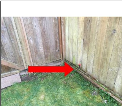
Image of wood rot along bottom of fence.
