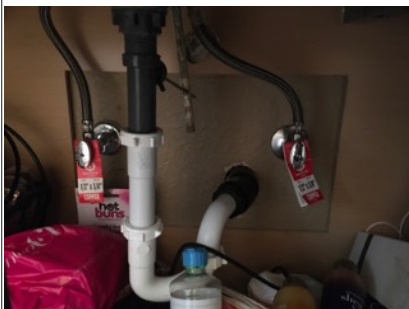
Image of plumbing under sink
