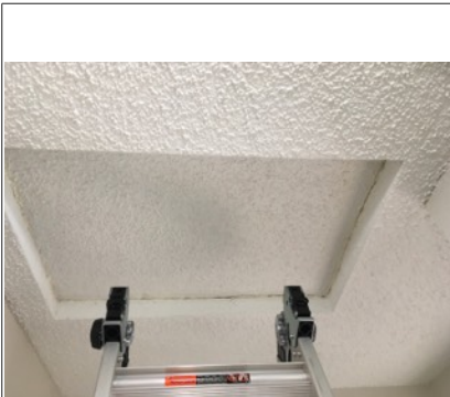
Access hatch to attic outside master bedroom
