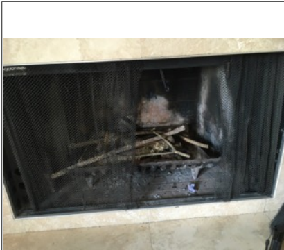
Image of fireplace with mesh screens
