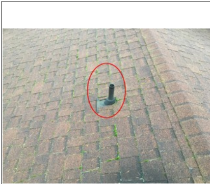
View of plumbing vents.
