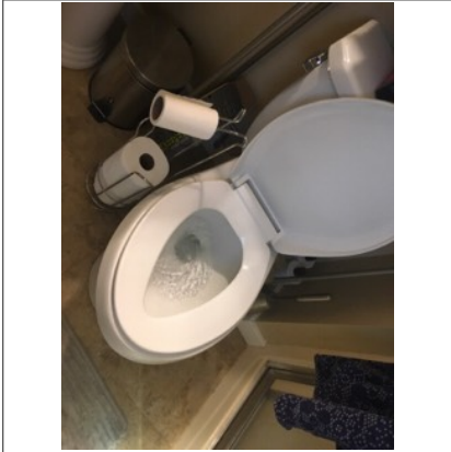
View of toilet with running water
