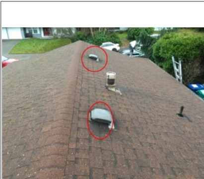
View of roof vents
