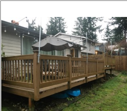
View of deck
