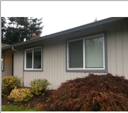
View of T-111 siding
