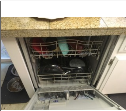
Dish washer was tested and is functional at time of inspection.
