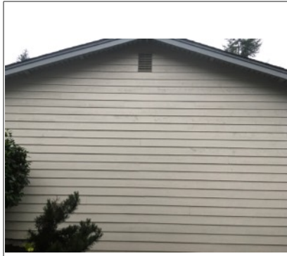
View of wood siding.
