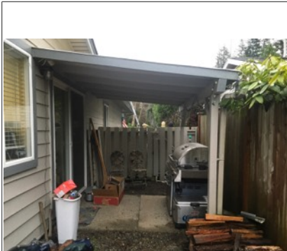
View of porch cover.
