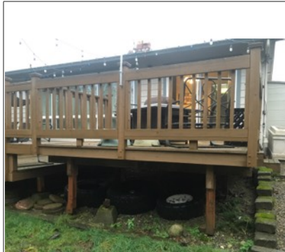
View of deck
