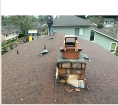
View of roof
