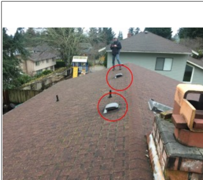
View of roof vents
