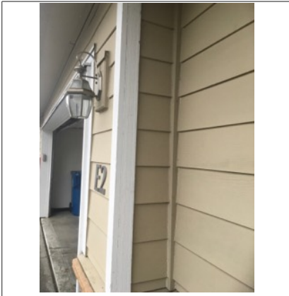
View of wood trim.
