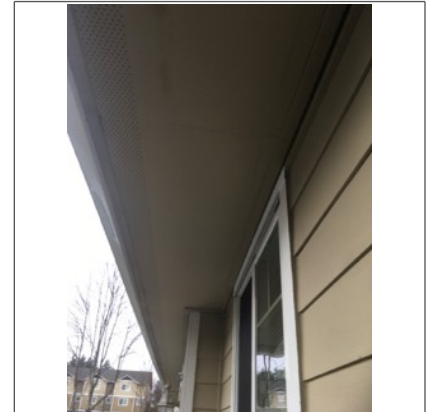
Image of soffit vents
