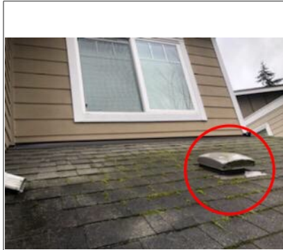
Image of roof vent
