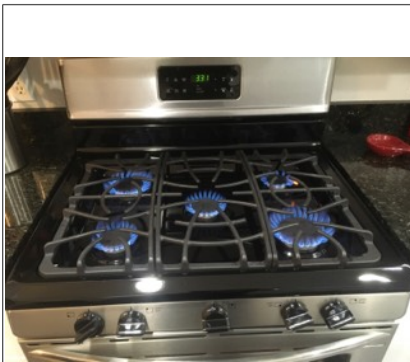
View of range with all burners functional.
