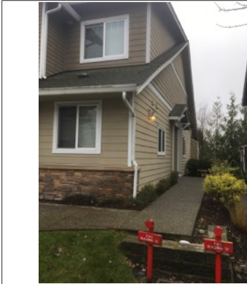
View of side of residence.
