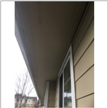
View of soffit and vents.
