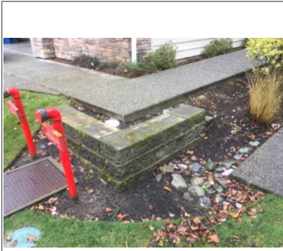
View of retaining wall on front of property.
