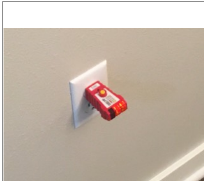
View of tested receptacle in dining room.
