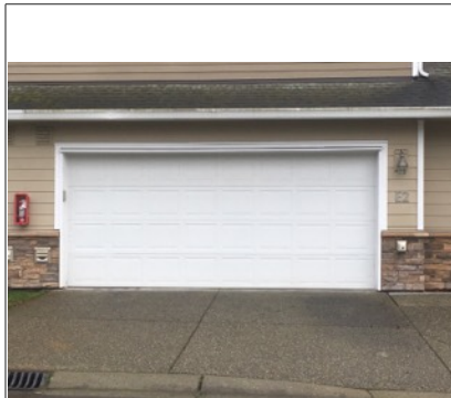
View of exterior garage door
