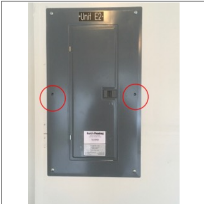
Missing two dead front panel screws. Further evaluation/repair by licensed electrical contractor.
